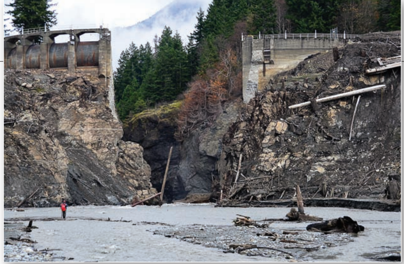
▲ Figure 1.1 Dam removal for river restoration. Removal of Glines Canyon Dam on the Elwha River, Washington, began in November 2012 to restore river ecosystems. [Brian Cluer/NOAA.]
